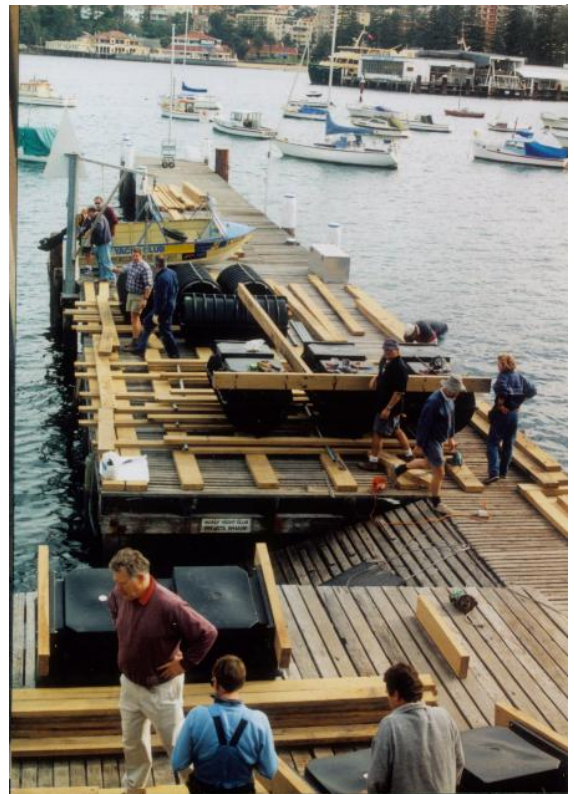
Assembly of the pontoon on the wharf
