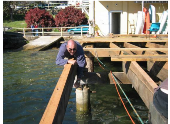
Current President Davis Lewis, tightening a few bolts on the wharf prior to the pontoon project
